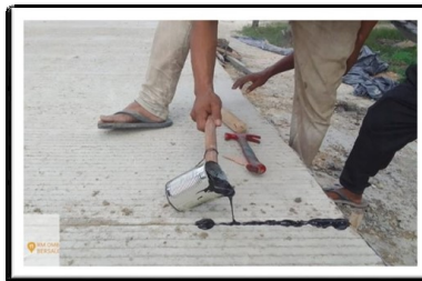
Gambar 4. 20 Proses Joint Sealant
