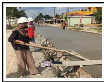
Gambar 4. 14 Proses Grooving
