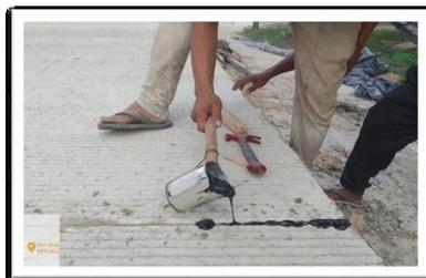
Gambar 4. 20 Proses Joint Sealant
